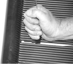
**5.** Push the plastic repair plug firmly, all the way down into the repair sleeve.
