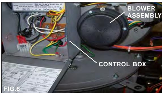
6. Route the terminal ring through the rear plastic grommet located inside the control box. (Fig. 7).
