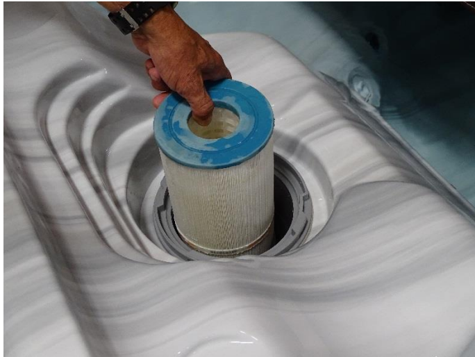
Figure 16. Drop in filter removal
